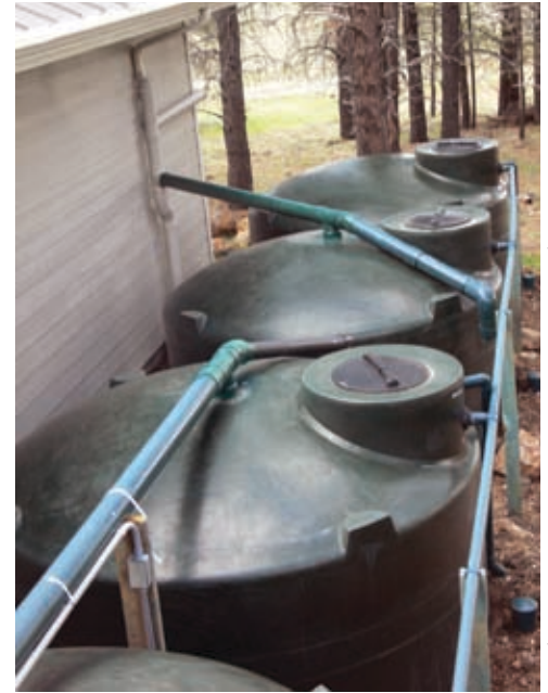
Rainwater catchment harvests all water, potable and irrigation, used by the home.
