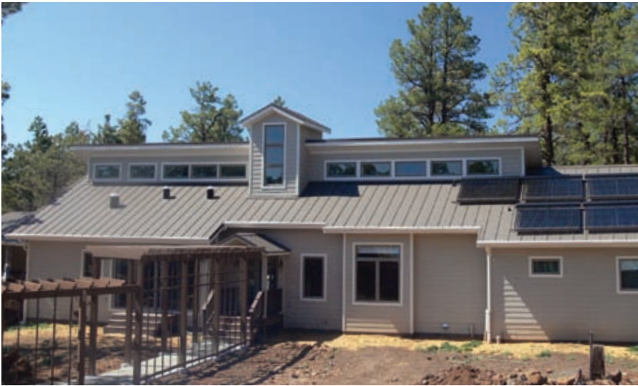
The home features a passive cooling tower (center of structure) and clearstory glass for passive thermal gain. The solar thermal system can also be seen on the roof to the right.
